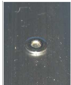
Outside hole with aluminum eyelet
