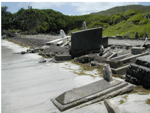
Fig. 4 Erosion of historic cemetery on Carriacou along the northeast part of the island. Sand mining at this site was stopped after public outcry
